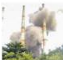
Smoke billows from a fire after an explosion in Neyveli Lignite Corporation power plant. PG/PTI
